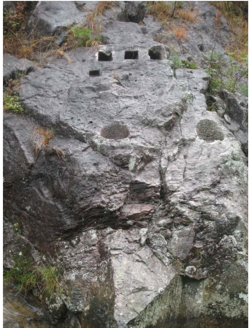
Hewn sockets in the stone abutments for precursor bridges adjacent to Santiao Bridge
