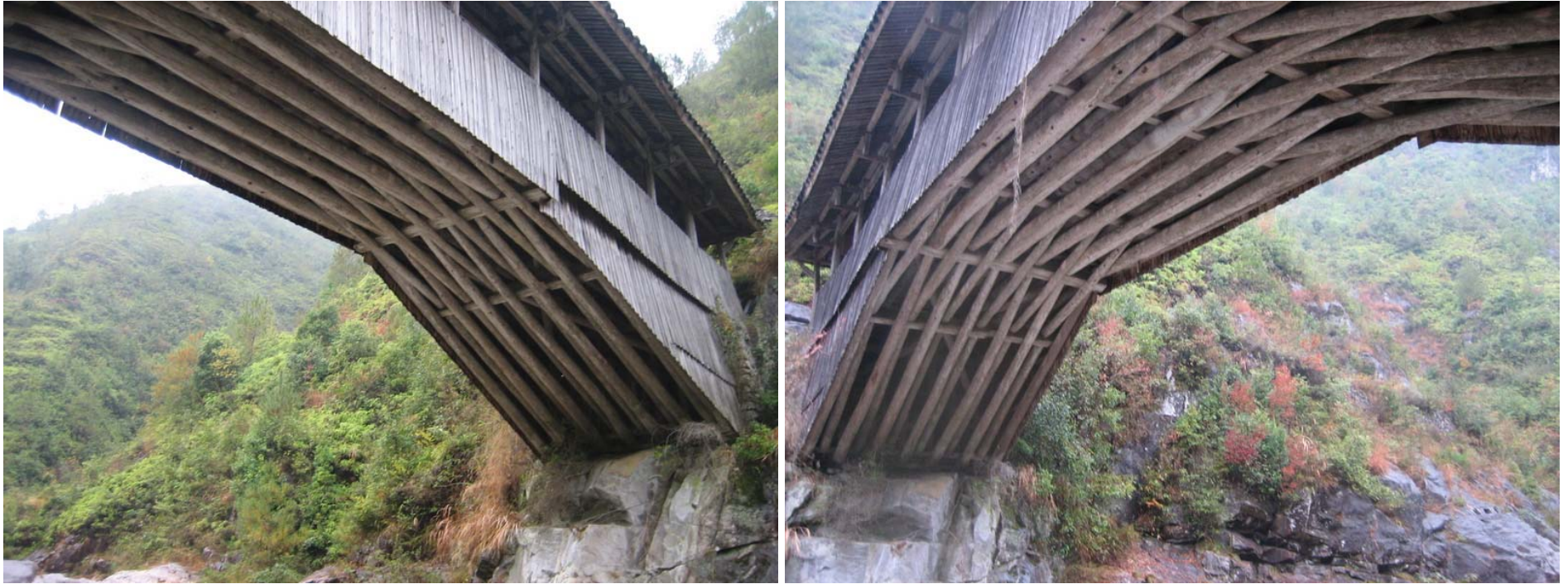
Santiao Bridge, Taishun County, Zhejiang Province Built in 1843. 32 meters long with a span on 21.26 meters. Width of 3.96 meters & height of 9.5 meters
