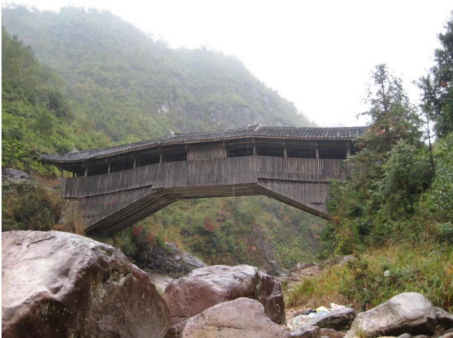
Santiao Bridge, Taishun County, Zhejiang Province Built in 1843. 32 meters long with a span on 21.26 meters. Width of 3.96 meters & height of 9.5 meters
