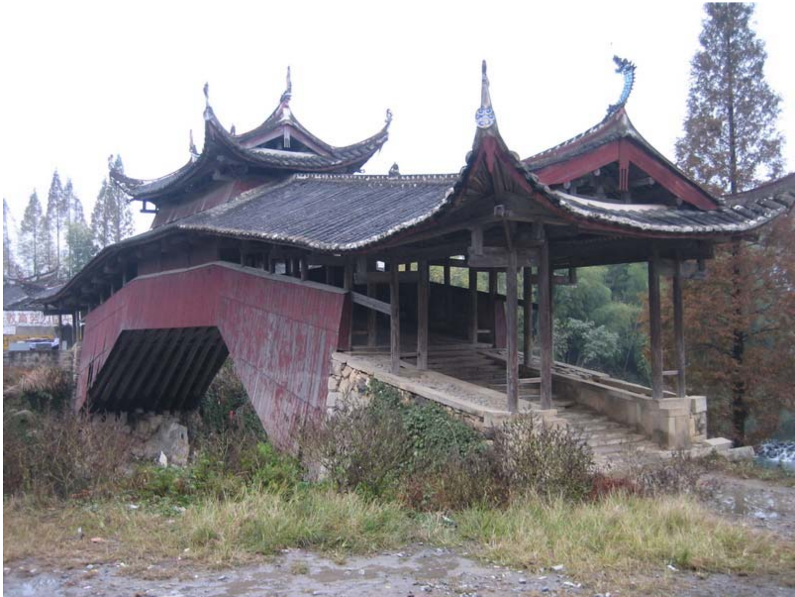
Xidong Bridge, the upstream 'sister' of Beijian Bridge (about 200 meters away), is 41.7 meters long and 4.86 meters wide with a span of 25.7 meters. First built in 1570, it was refurbished in 1745 and then repaired in 1827.
