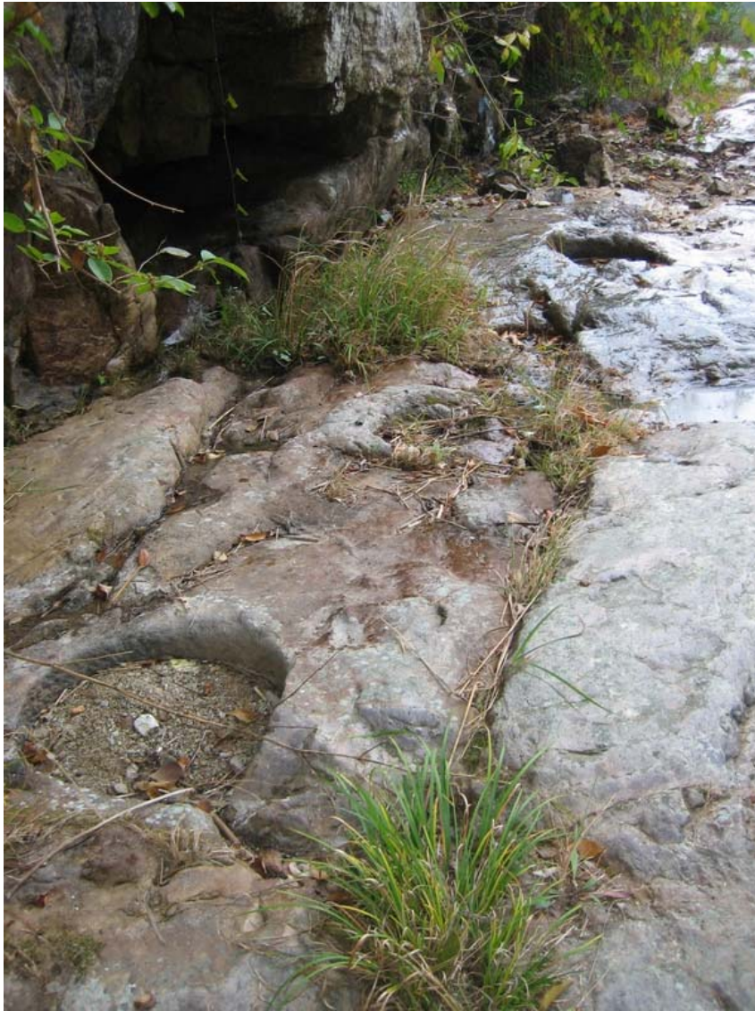
Hewn sockets in the stone abutments for precursor bridges adjacent to Santiao Bridge
