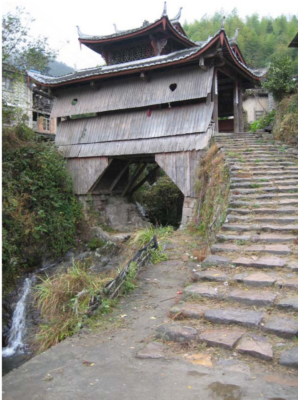
Baiyun Bridge, Jushui Township, Qingyuan County, Zhejiang Province Built in 1600s. Corridor is 8.34 meters long, 3.72 meters wide. Open span is 5.75 meters
