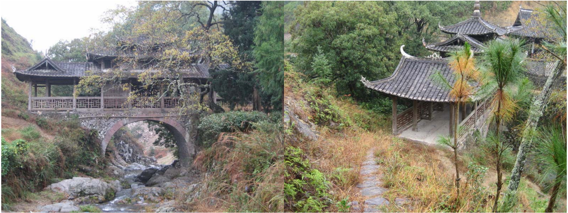
Yuewen Bridge, Zhoubian Village, Zhouling Township, Taishun County, Zhejiang Province Built in 1839. 22.9 meters long, 4.15 meters wide, with a single span of 7.6 meters
