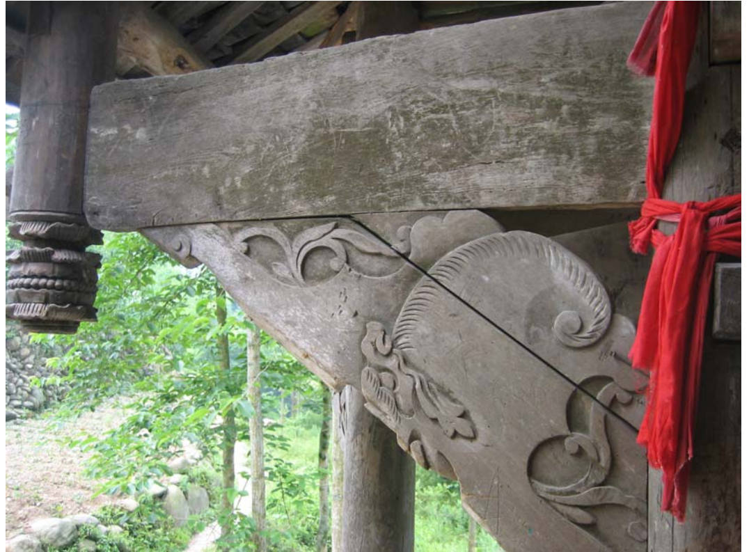
New and old wood used in the restoration
