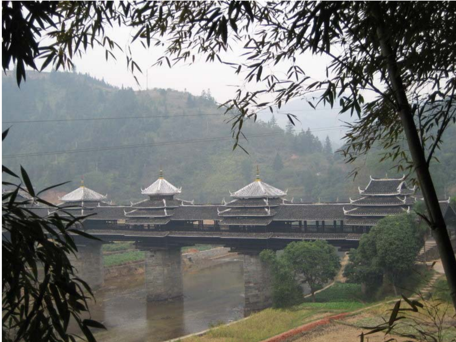
Chengyang (Yongji) Bridge, Linxi Township, Ma'an Village, Sanjiang, Guangxi Zhuang Autonomous Region Begun in 1912 and completed in 1924. Sections destroyed by flood waters in 1937 and 1983 77.76 meters long, 3.75 meters wide. 3 piers. The pavilions rise 11.52 meters above the stream.
