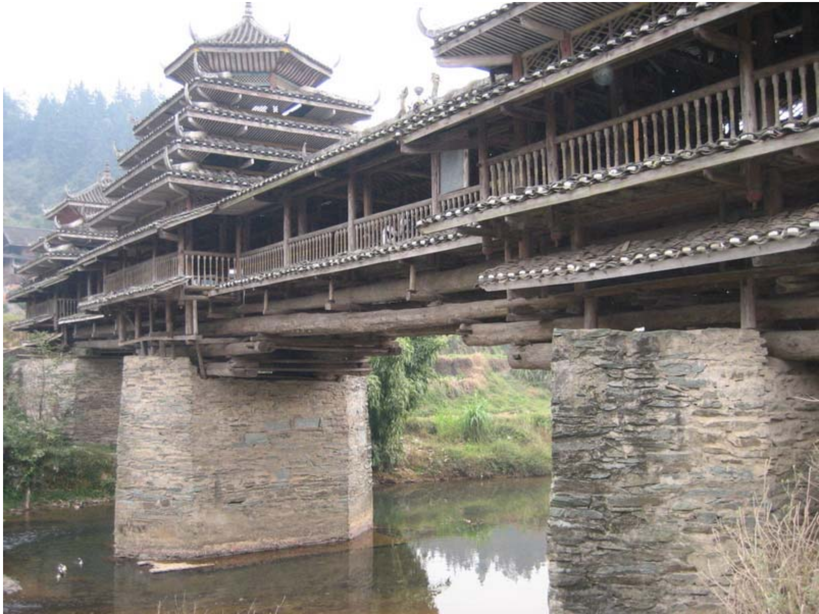
Cantilevered Beam Structure of Bajiang Bridge
