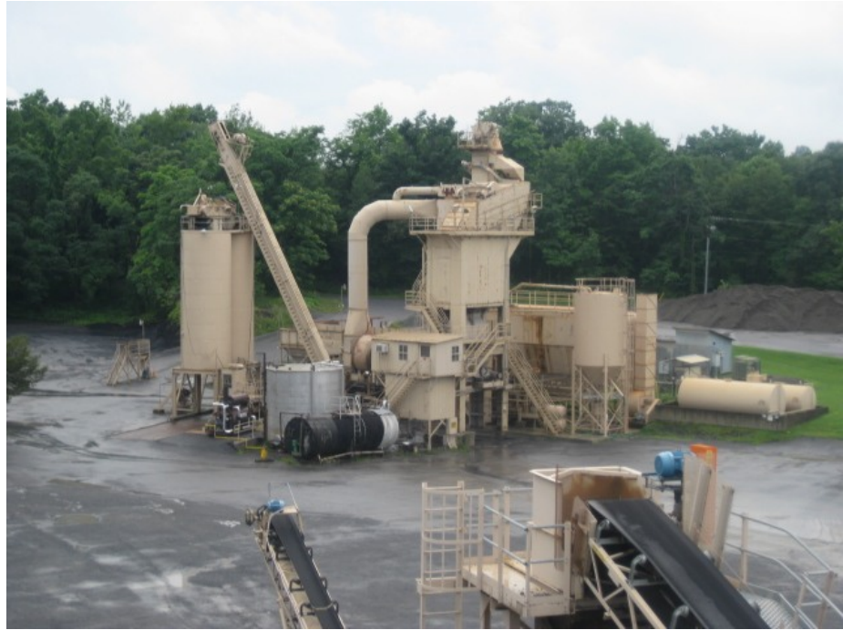
Figure 20. Photo showing blacktop plant at Colarusso quarry on Becraft Mountain.
