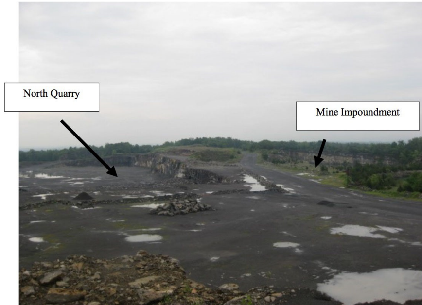
Figure 24. Photo showing differing elevations of mine impoundment surface (260 feet asl) on right and dry North Quarry floor (235 to 245 feet asl) on left.
